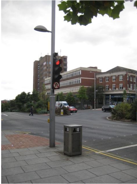
Figure 6 Combined traffic signal with lamp post
