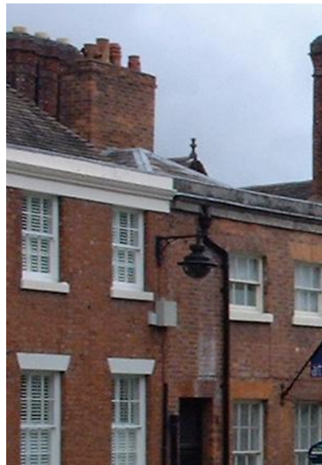
Figure 5 CCTV camera disguised as an historic wall lamp
