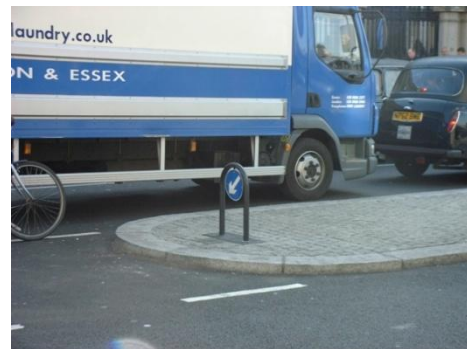
Figure 6 Keep left signs are not compulsory. Where they are used (where it may not be clear that vehicles should keep left e.g. after a break in a central reserve), then bright yellow/orange panels are not a requirement.
