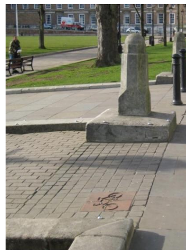
Figure 7 Paving inset cycle route sign
