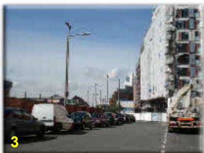
Loop diverted along north side of Brewery as part of long term planning of the site
