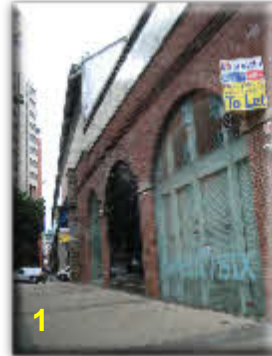
Area where a high level walkway could link the present footbridge to the Sovereign St site
