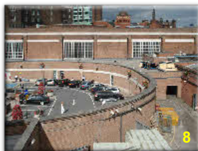
Area for new Station exit from footbridge and pick up / drop off area
