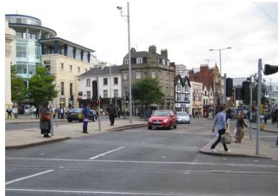
Figure 2 Complex and busy town centre pedestrian crossings can do without guard rails – here a double kerb helps steer less mobile pedestrians to the controlled section.
