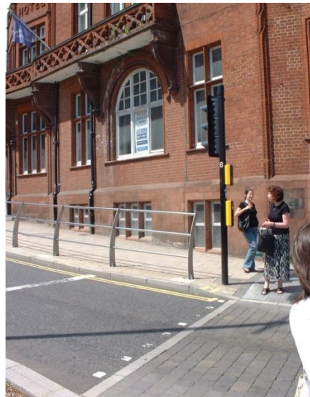
Figure 5 A simpler guard rail type in a city centre mixed priority route scheme - allows good visibility
