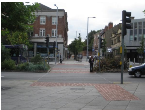
Figure 10 Inner urban ring road where an underpass has been replaced by a straight surface crossing without guard railing
