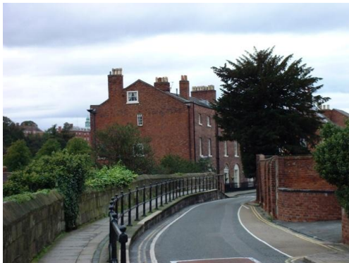
Figure 6 Historic railing should be retained
