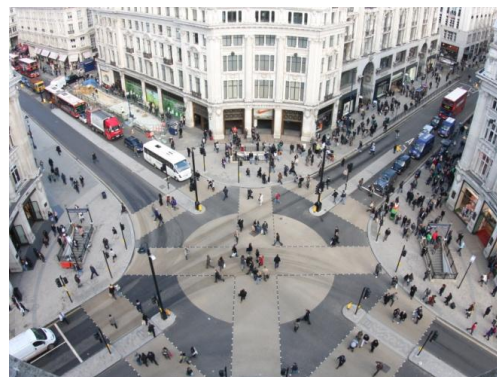
Figure 7 A busy guard rail free city junction with maximum capacity for easy pedestrians movements where until recently it was fully guard railed Photo ©Atkins, by kind permission
