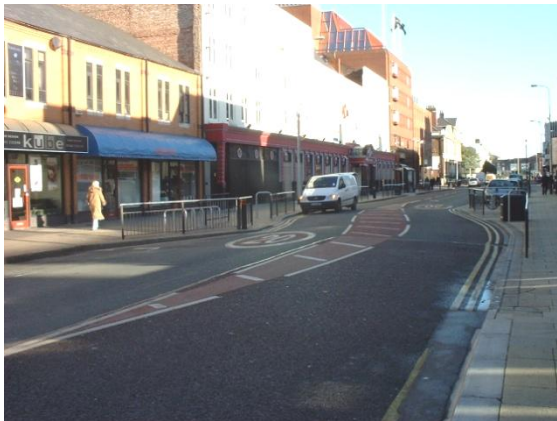
Figure 4 Guardrail used unnecessarily as fencing to cycle stands and to emphasise a chicane
